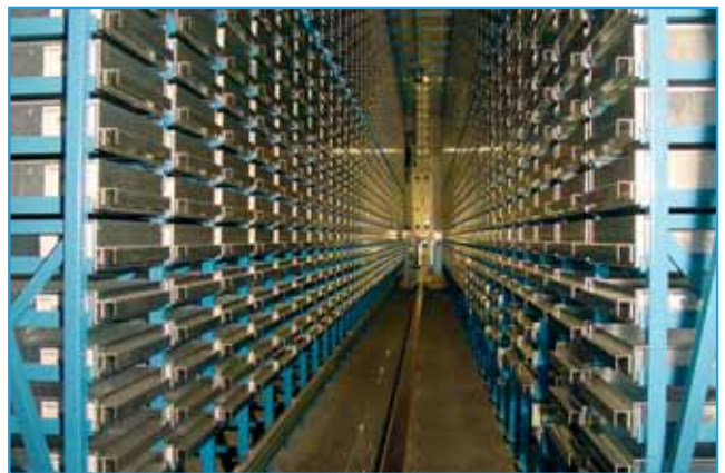
Inside the warehouse showing boxes handled by automated robots
